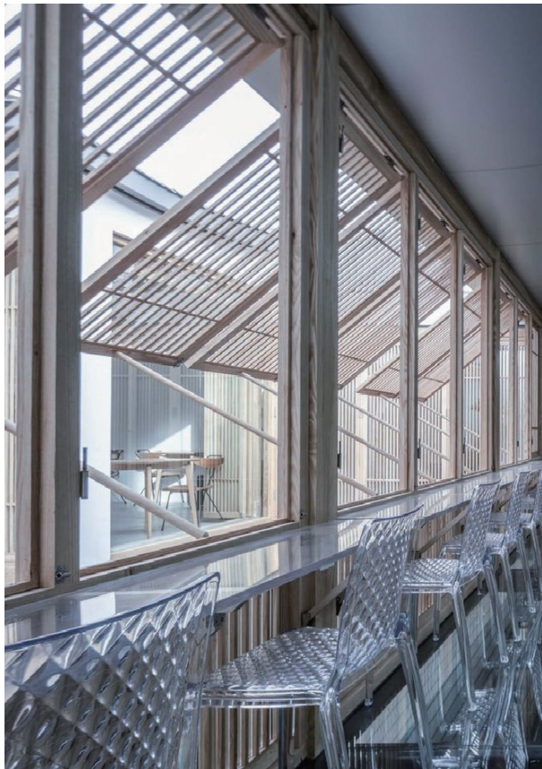
supported by simple oblique brace and opened horizontally
