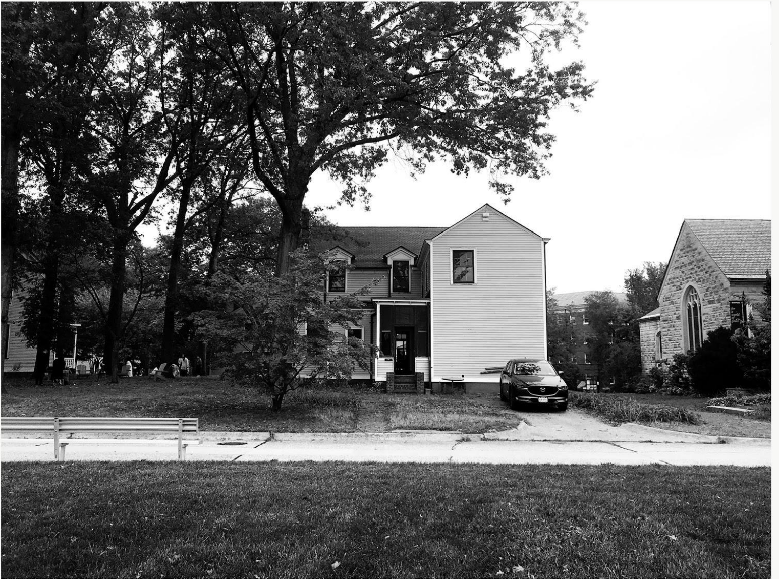
The site for intervention on House 14 is the prototype for distributed water.
