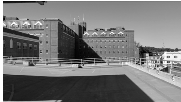
Rooftop of parking garage
