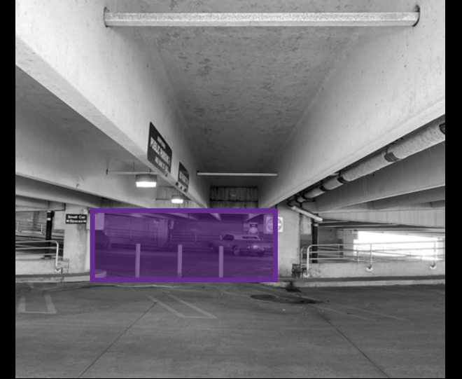
In between levels - Blocked to cars
