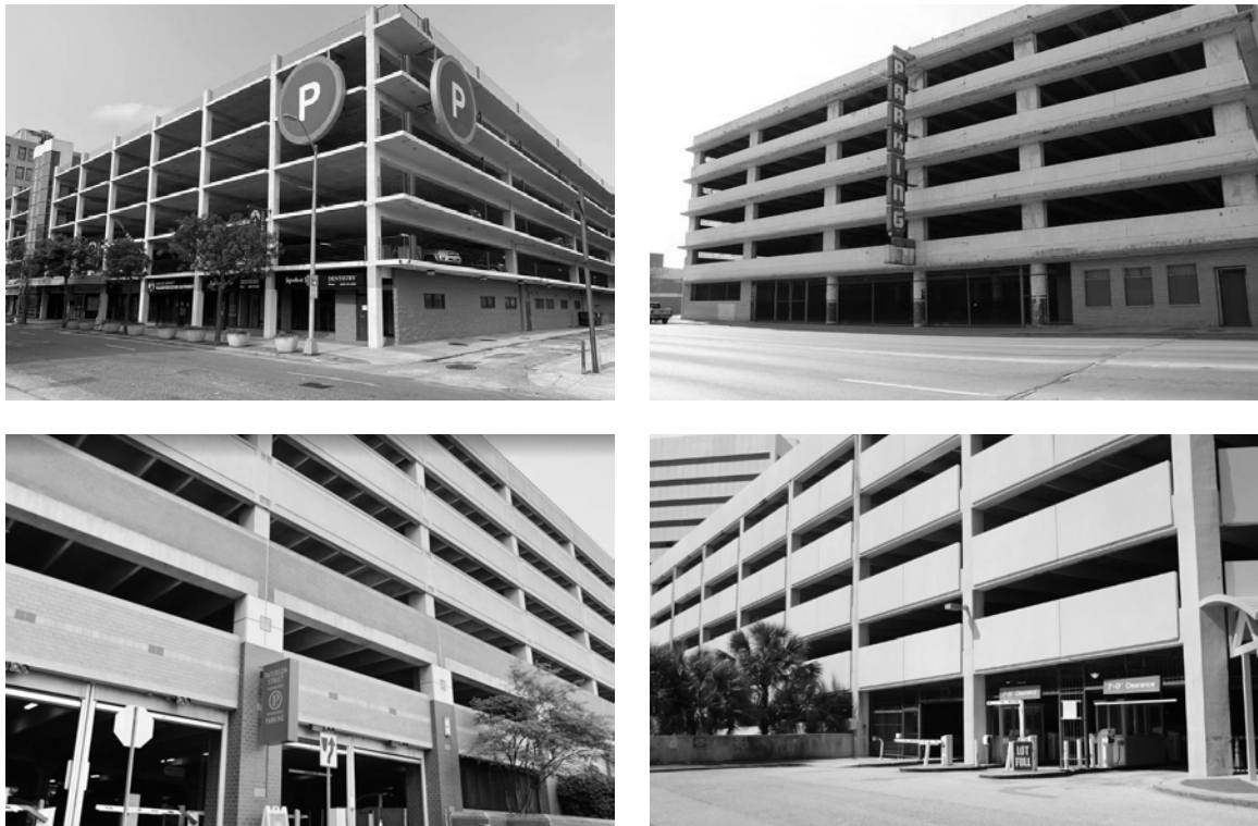
Examples of other generic parking garages that the thesis' strategies can be employed within. (Top Left: Atlantic City Parking Garage NJ, Top Right: Knightley's Parking Garage NJ Bottom Left: Patterson Street Parking Garage NJ, Bottom Right: Water-Street Parking Garage NJ)
