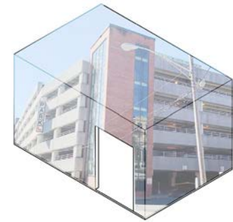
PARKING GARAGE EXTERIOR
