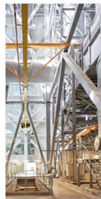
Waste to Energy
